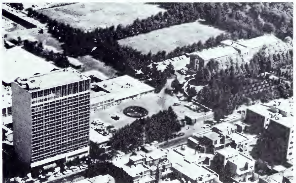
An aerial view of the U.S. Embassy compound in Tehran prior to its seizure and occupation in November 1979. (Department of State photo)
